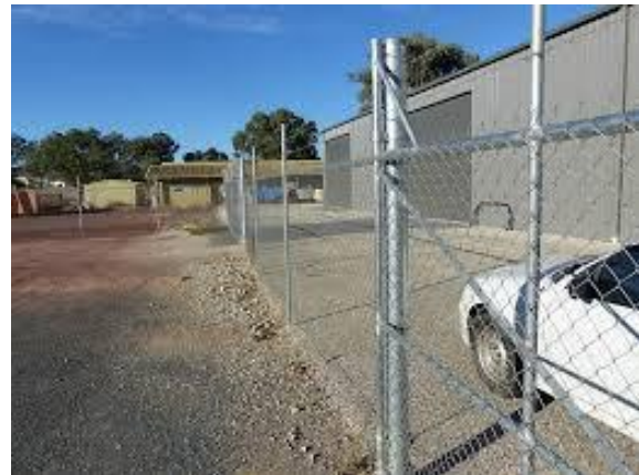
Typical barbed wire topped “chain-link” perimeter fence
