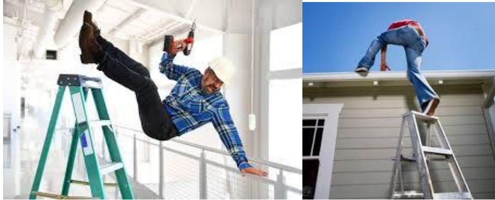
Unsafe use of ladders
