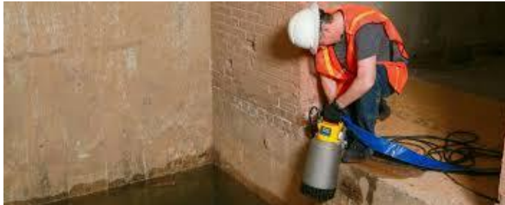
A worker retrieving a submersible pump
