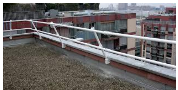
Fixed roof parapet handrails
