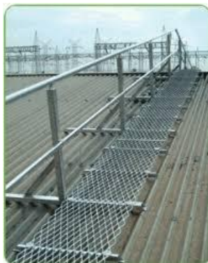
Roof top maintenance walkway
